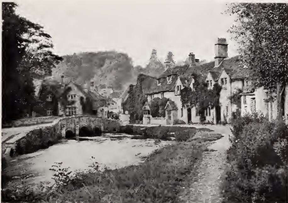
Illus. 86.—View showing informal development.
